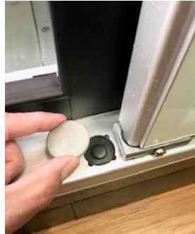
撬出塑料盖 Remove Plug Cap
