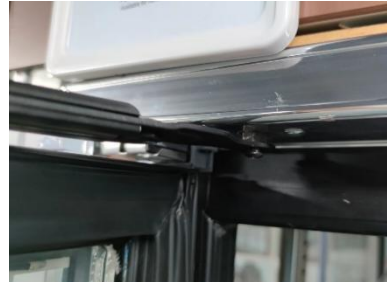
拧紧限位板螺丝 Tighten Hold-Open Screw
